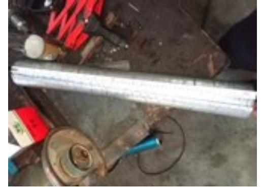
Sheet rolling and riveting
